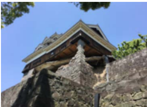
The damage of Kumamoto castle
